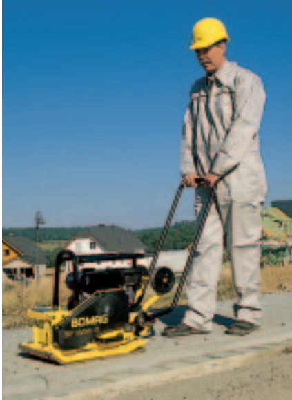
Compacting paving blocks with vulcolan mat
